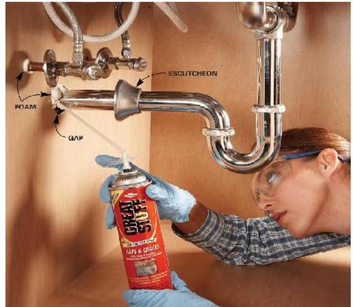
Pull back the escutcheons on plumbing pipes where they enter exterior walls and you'll probably see generous gaps around the pipes. In cold weather, you might also feel the draft coming in. All it takes is a can of expanding foam to seal those leaks.
