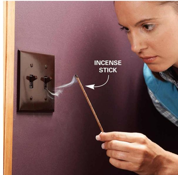
Locating air leaks can be tricky. They're often so small as to be hardly noticeable. To find them, follow a trail of smoke. Close all the windows in the house, turn off all the fans and exhaust fans, and shut off the furnace. Light some incense and walk slowly around the outer walls of the house. Anywhere you notice the smoke blowing away from something or being sucked toward something, there's probably an air leak. Now that you've found it, seal it!
